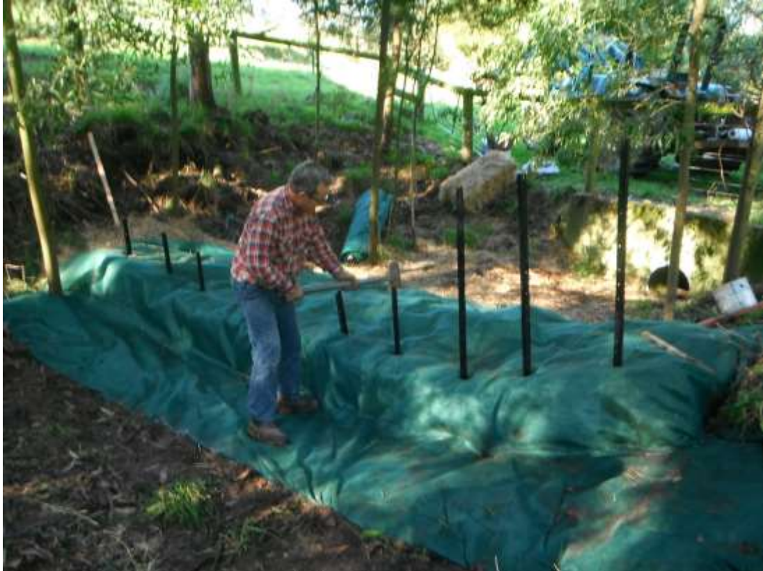
Figure 5: Method 1. Hay bales staked down and covered with shade cloth
