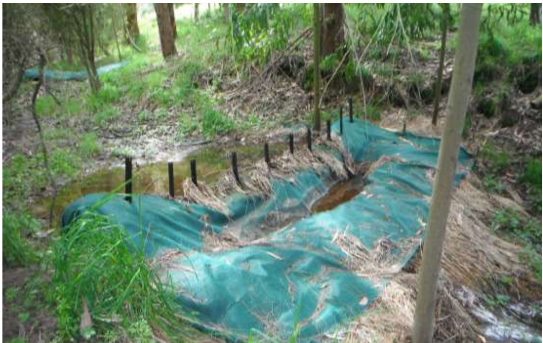
Figure 13: The heavier rain events overwhelmed the sediment traps and they were found to be largely ineffective under such conditions
