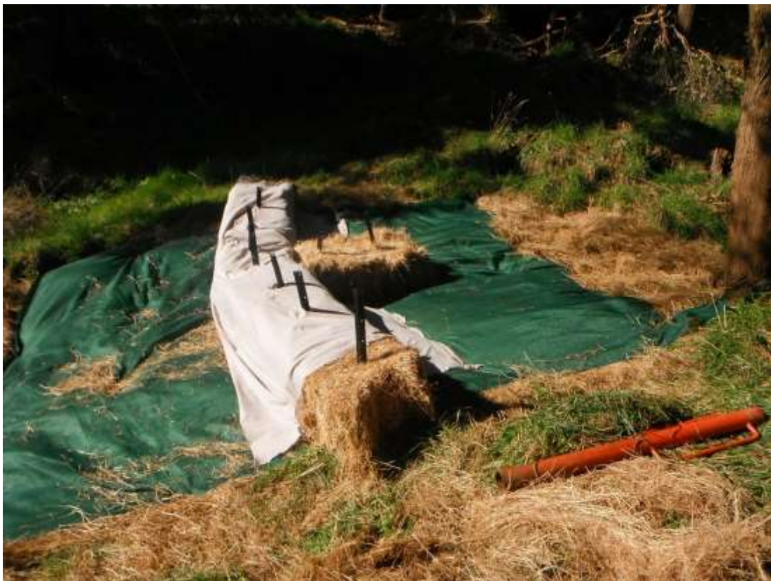
Figure 6: Method 2. Shade cloth covering a thick layer of hay with bales staked down and covered in a geotextile
