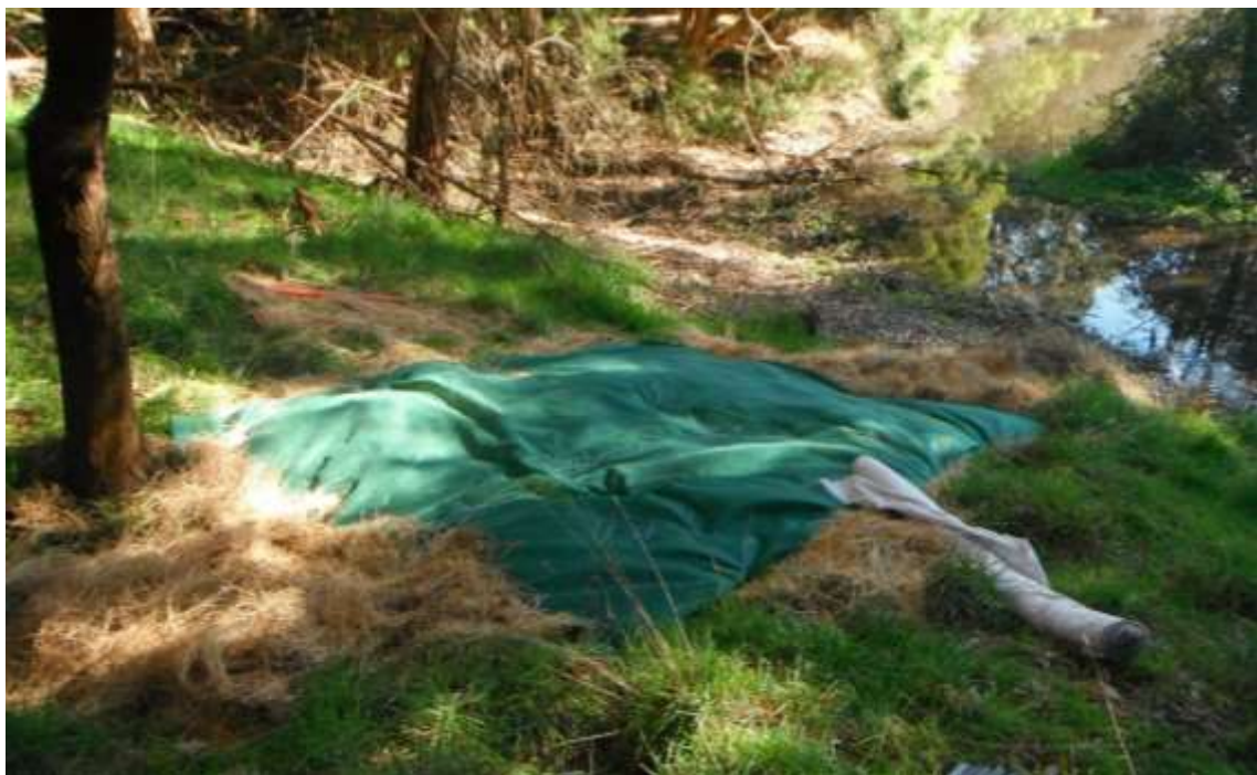
Figure 16: the preferred silt trap design method
