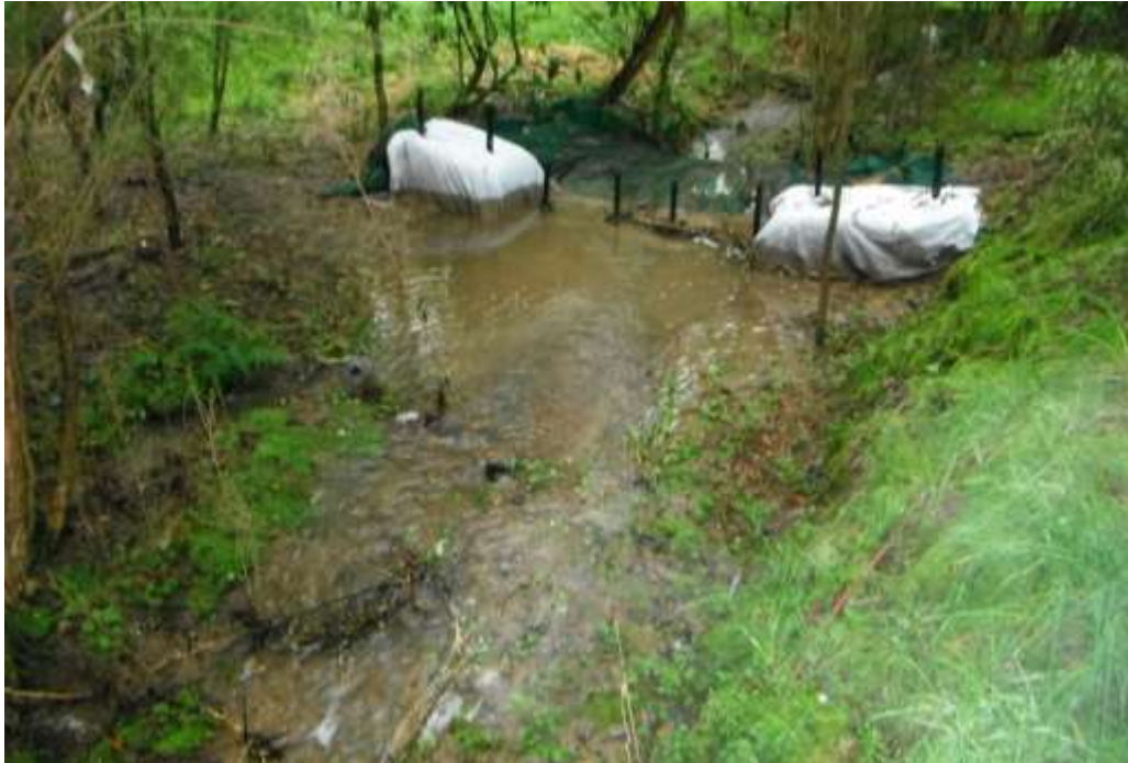
Figure 14: Another example of the heavier rain events that overwhelmed the sediment traps and they were found to be largely ineffective under such conditions
