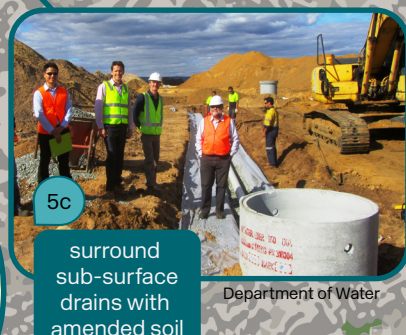
5c surround sub-surface drains with amended soil
